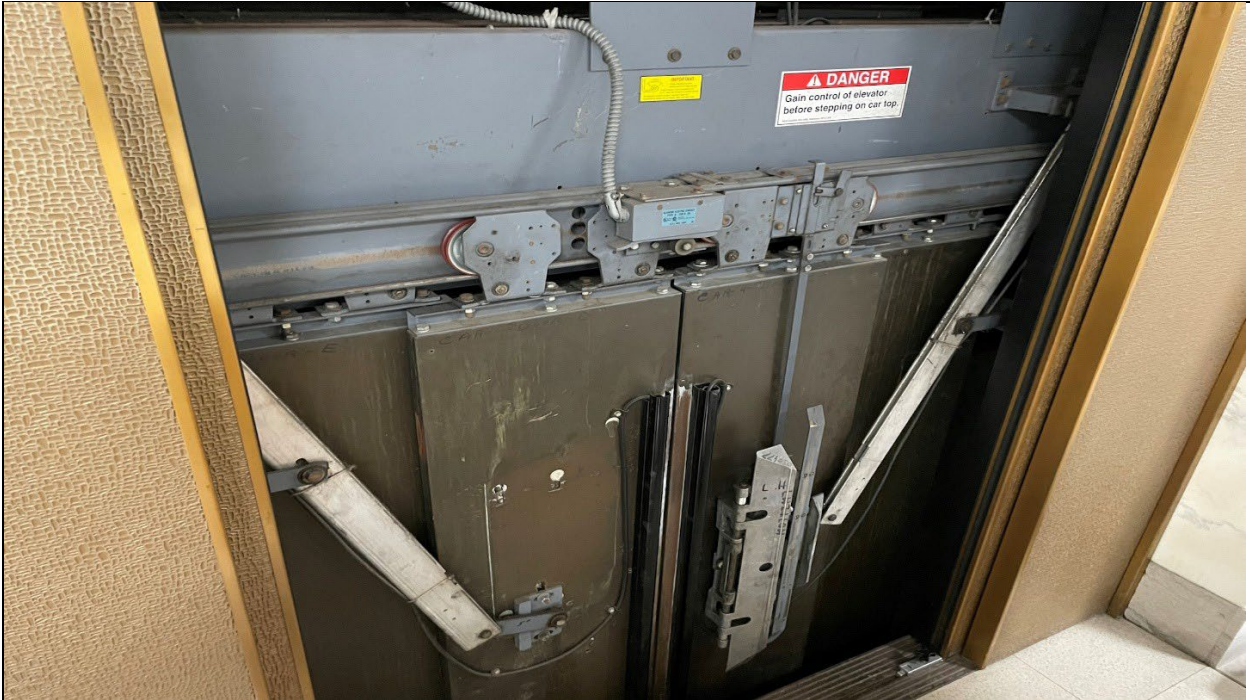
Photograph 7. Side of elevator car.
