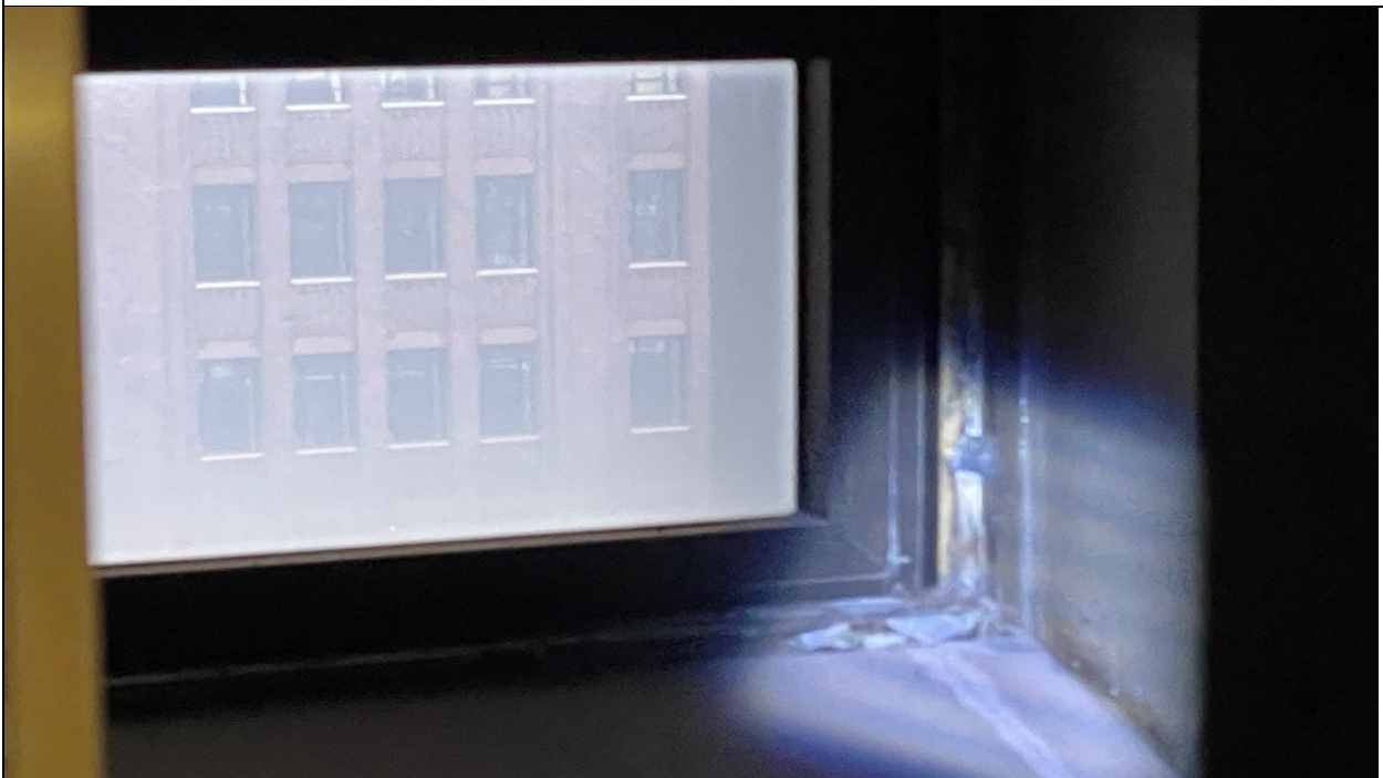
Photograph 10. HA-5, Window Frame Caulk, Hoistway Windows (assumed ACM).
