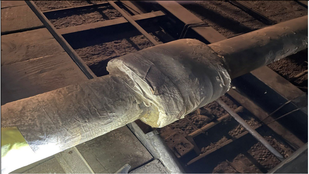
Photograph 13. HA-3, Pipe Fitting, Elevator Penthouse Crawlspace Steam Pipe
