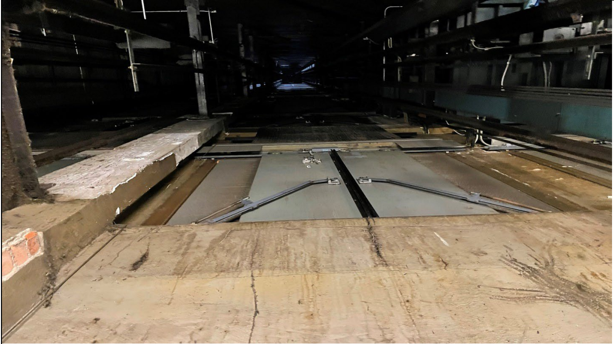
Photograph 5. Vertical view of hoistway from pit level looking up.
