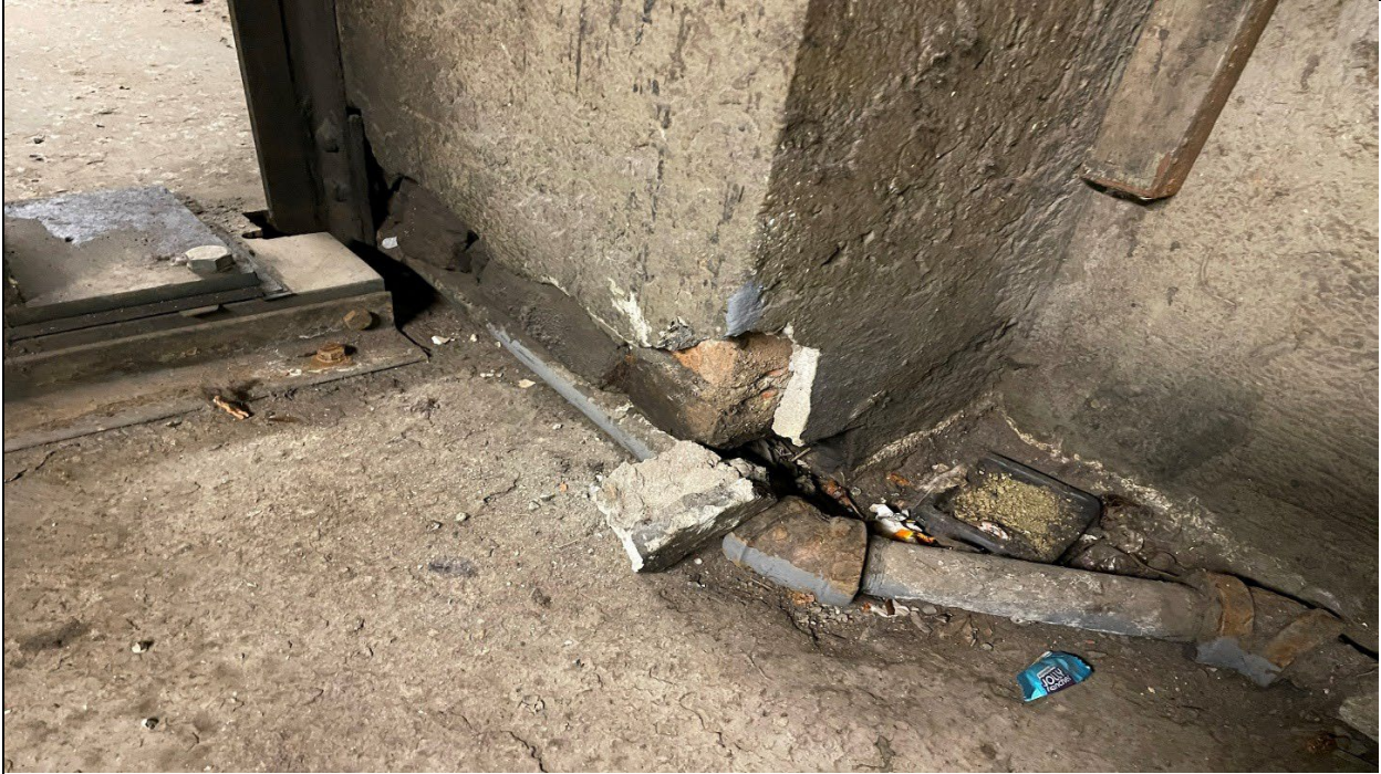
Photograph 3. HA-1, Plaster/Mortar from elevator pit walls.
