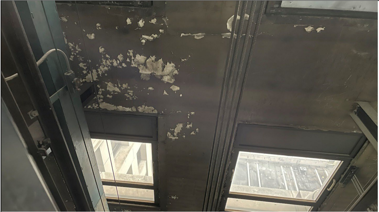
Photograph 9. Hoistway from upper floors.
